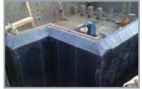
Post-applied bitumen based waterproofing for floors and walls can be easily installed using Proofex self-adhesive membranes in conjunction with Proofex Protection Board PP or Proofex Sheetdrain 81 .
