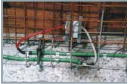
Supercast Predimax injection hose waterstops for future provision of sealing leaking joints.
